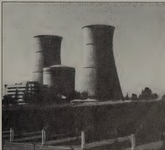
Solar panels surround Sacramento Municipal Utilities District’s defunct nuclear power plant. —ECO-PIONEERS
